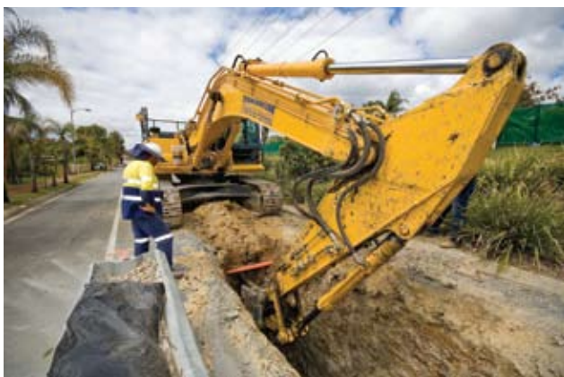
Above: Constructing within a road on Southern Regional Water Pipeline
